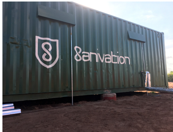
FIGURE 7: SHIPPING CONTAINER HOUSING THE TREATMENT PLANT
